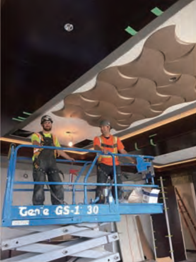
Ceiling in Lobby
