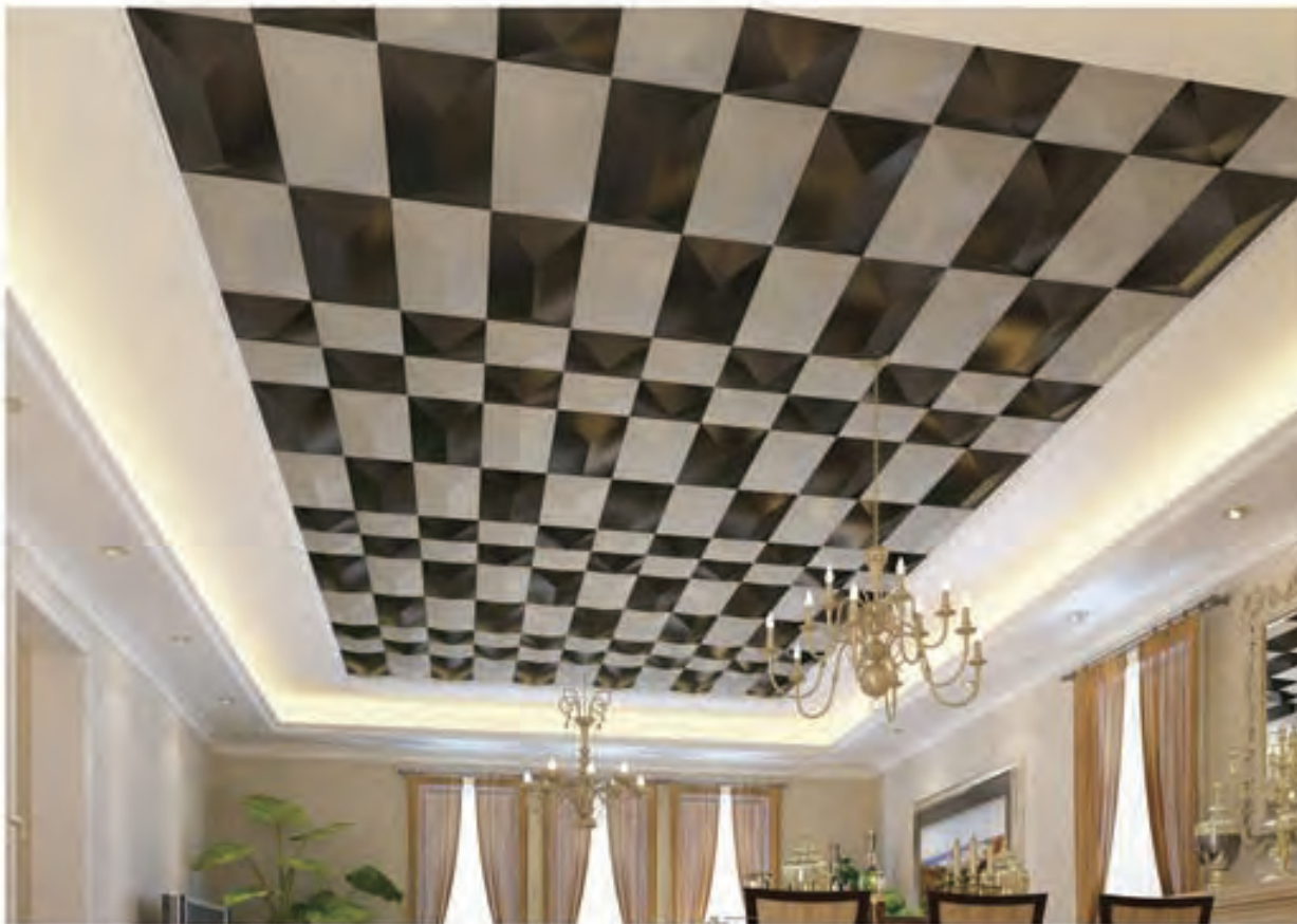
Living Room Ceiling
